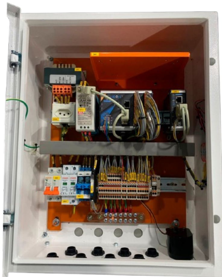
Figura 1 - Painel ACOS500 BM STD com Gateway Modbus
